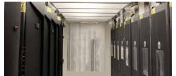
Cabinet Supported Cold Aisle Containment
