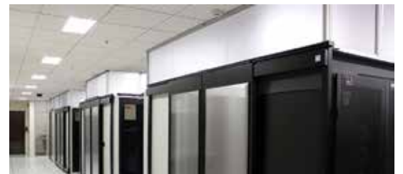
Floor Mounted Hot Aisle Containment
