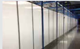
“Light Box” Containment
