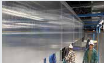
Installation of SPS
